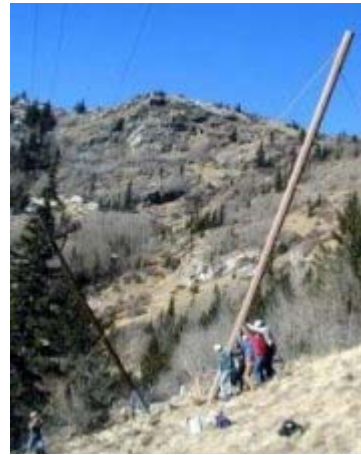
b) Composite pole installation
